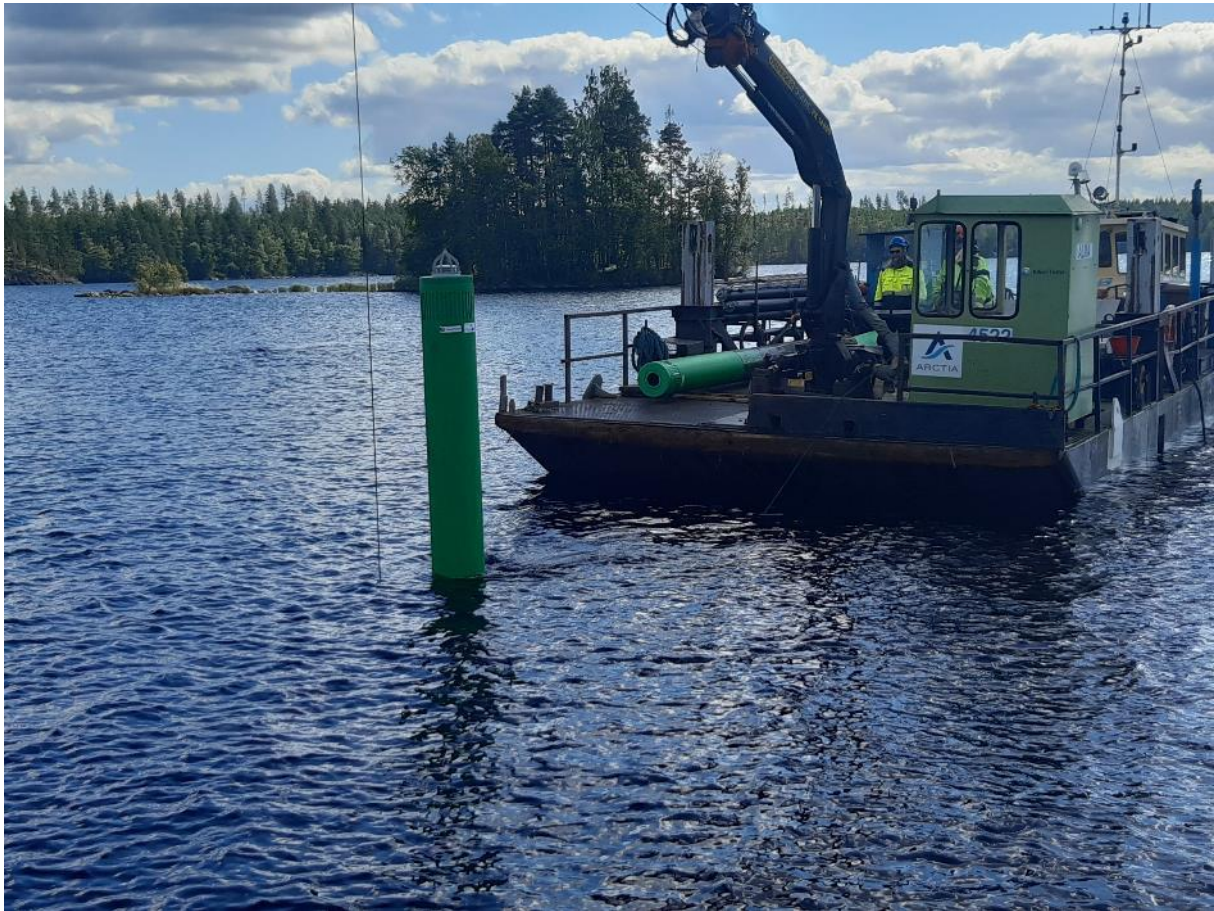
Figure 7: A Smart buoy being installed on the pilot fairway
