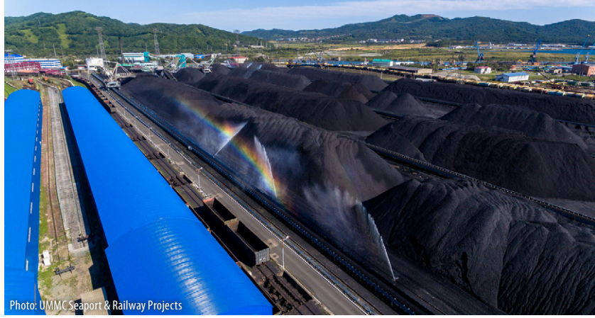
Photo: UMMC Seaport & Railway Projects
